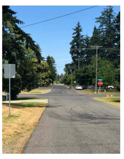
Current site conditions across Parkland do not provide a separated area for pedestrians and are generally characterized by a 55-foot right-of-way with 20-foot pavement widths.
